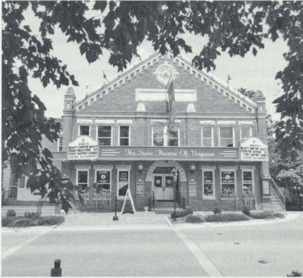
Sinking Spring Church of 1833. The old church constitutes the auditorium of the theatre. The front part is a later addition.
