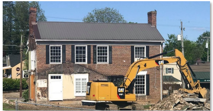
More recent additions to the original house have been removed to make it ready to be relocated.
